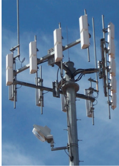
Figure 16.5 Sectorized base-station antenna.
